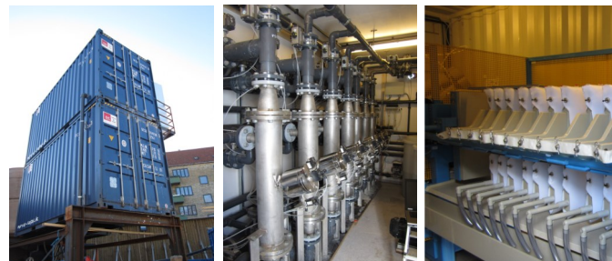
Picture 3: UF system in container (left) - LiqTech SiC membranes mounted in stainless steel housings (middle) - Filter press for sludge treatment (Right)
