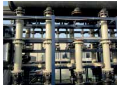
Textile Waste Water, Egypt: LiqTech's SiC membranes used for UF stage. Capacity: 70 m 3 /h.
